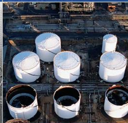
Mortar pools & Coal slurry tank, Butter storage tank & Stockyard
