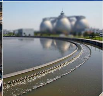
Pump house & collection well Biochemical reaction tank
